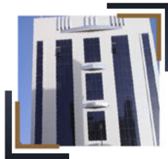
Cladding (A.C.P) Glass & Glazing Work
